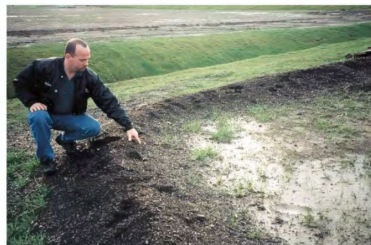
Compost berm to stabilize site.
