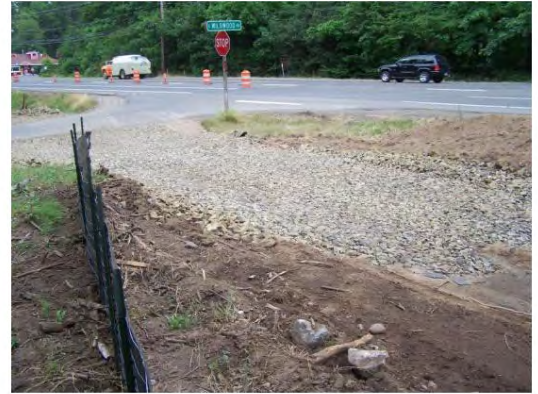
Gravelled site entrance.
